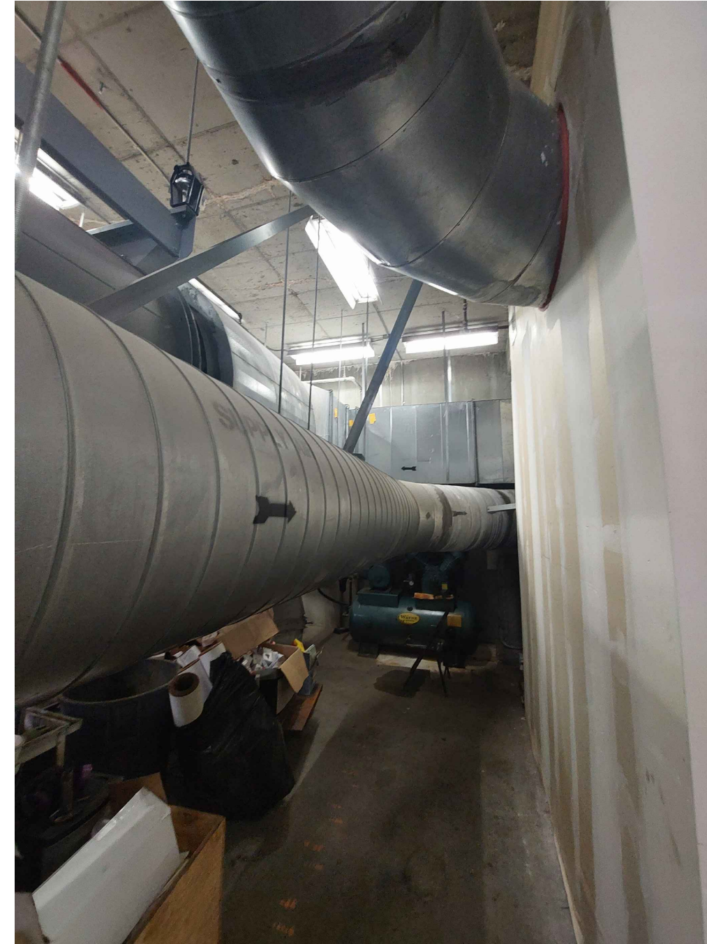
A PHOTO - SUPPLY DUCTS SCALE: 3/16" = 1'-0"
