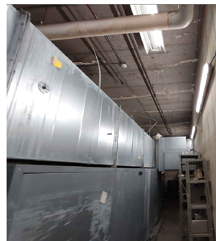
C PHOTO - FAN ROOM CEILING M2.04 SCALE: NONE
