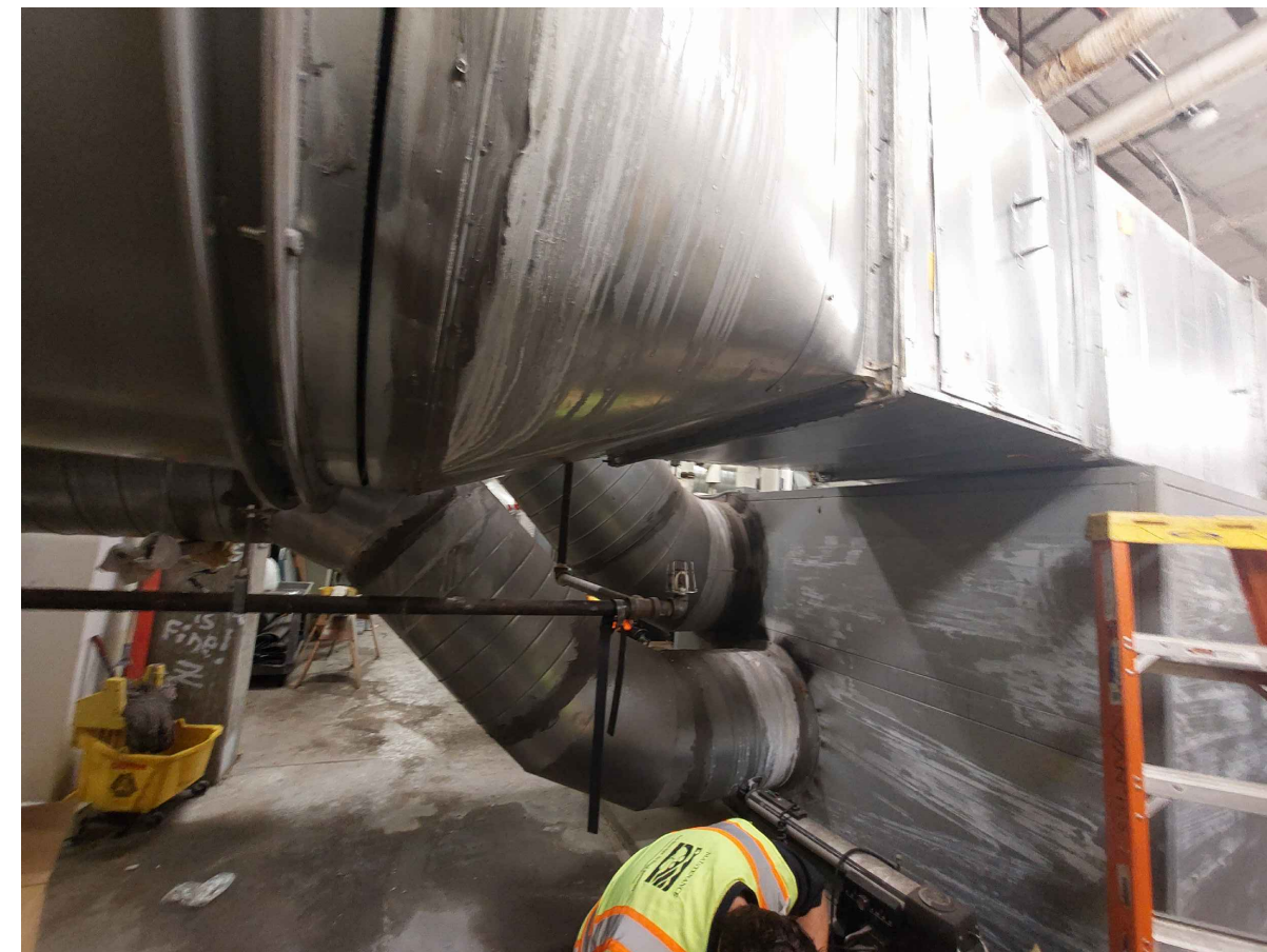
B PHOTO - AHU-2 & R/A DUCT SCALE: 3/16" = 1'-0"
