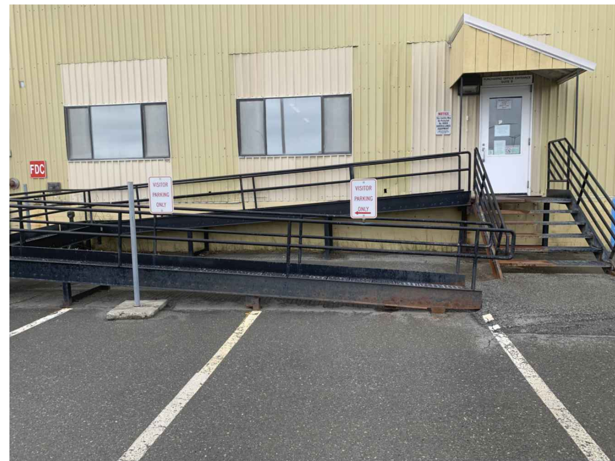
A DEMOLITION PHOTO 1 SCALE: NTS
