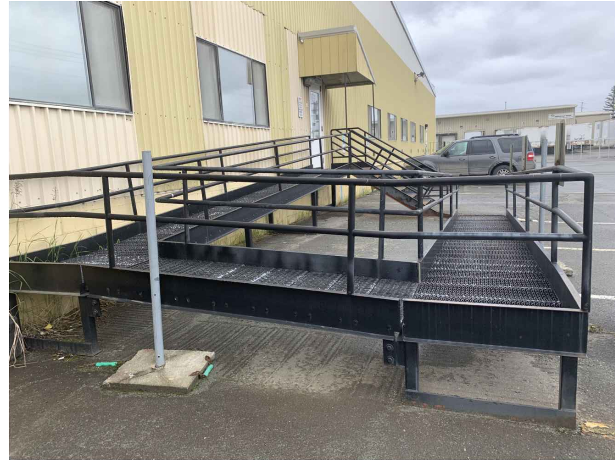
B DEMOLITION PHOTO 2 SCALE: NTS
