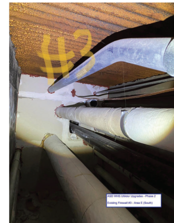
2 REFERENCE PHOTO FIRE WALL #3 A3.01 NTS
