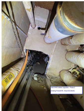
5 REFERENCE PHOTO FIRE WALL #5 A3.01 NTS
