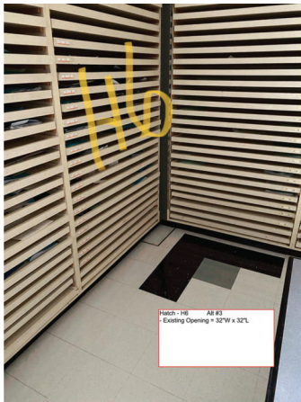
10 REFERENCE PHOTO ACCESS HATCH H6 A3.02 NTS
