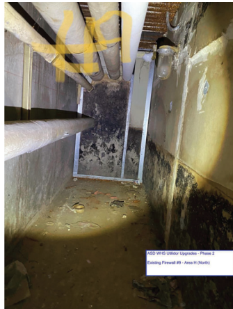
9 REFERENCE PHOTO FIRE WALL #9 A3.01 NTS
