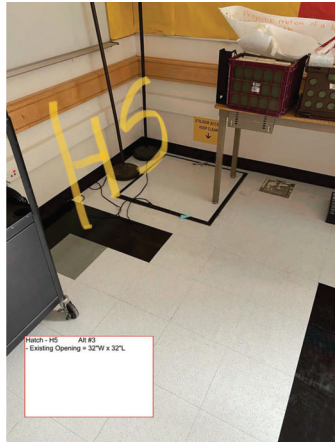
9 REFERENCE PHOTO ACCESS HATCH H5 A3.02 NTS
