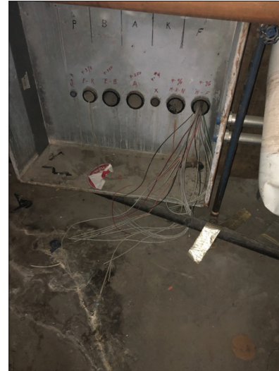
2 ABANDONED SPLICE BOX PHOTO NO SCALE
