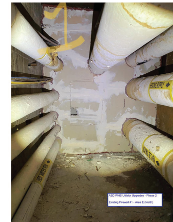
1 REFERENCE PHOTO FIRE WALL #1 A3.01 NTS
