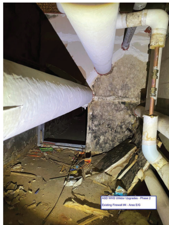
4 REFERENCE PHOTO FIRE WALL #4 A3.01 NTS
