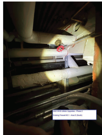
3 REFERENCE PHOTO FIRE WALL #3.1 A3.01 NTS
