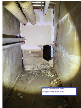
8 REFERENCE PHOTO FIRE WALL #8 A3.01 NTS
