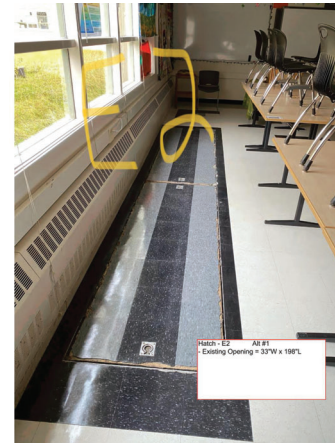
2 REFERENCE PHOTO ACCESS HATCH E2 A3.02 NTS
