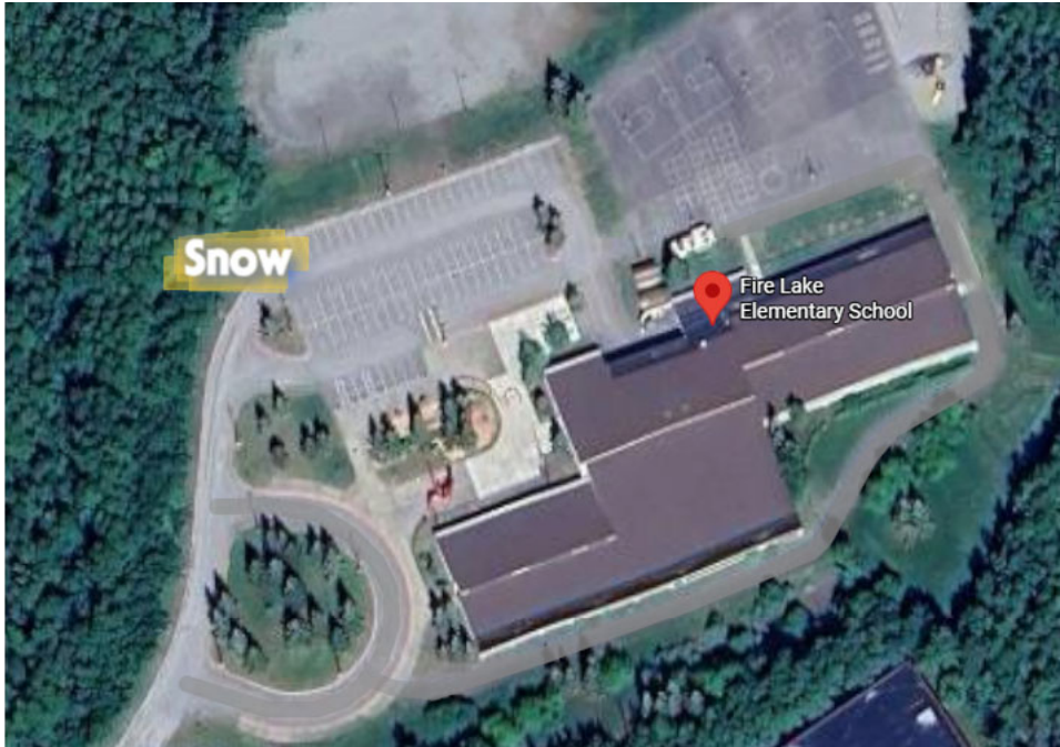
FIRE LAKE ELEMENTARY SCHOOL
