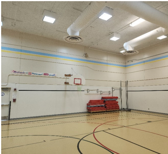
Figure C3. Gymnasium, Looking Southeast
