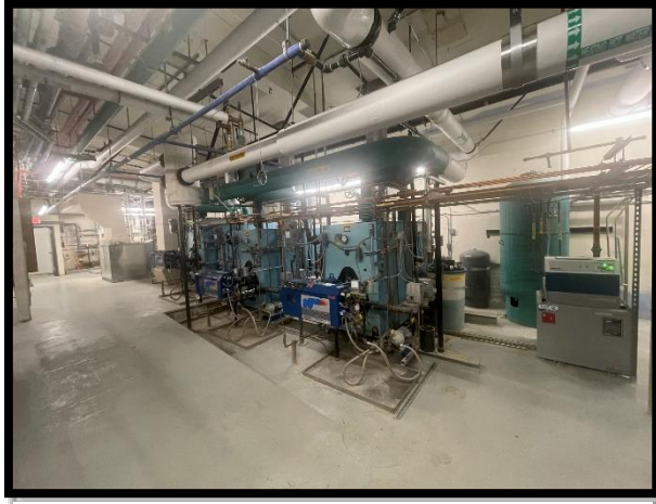
FIGURE 1. EXISTING BOILER ROOM
