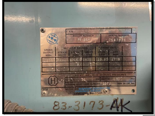
FIGURE 2. EXISTING BOILER SIZE
