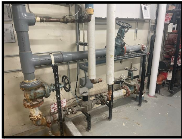
FIGURE 3. WATER SERVICE PIPING TO BE REPLACED
