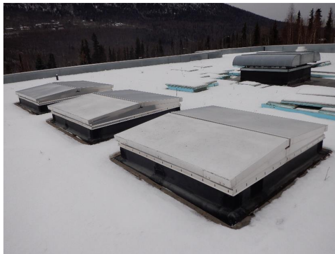
Figure 1 – Row of Smoke Hatches on Multipurpose Room Roof to be Removed
