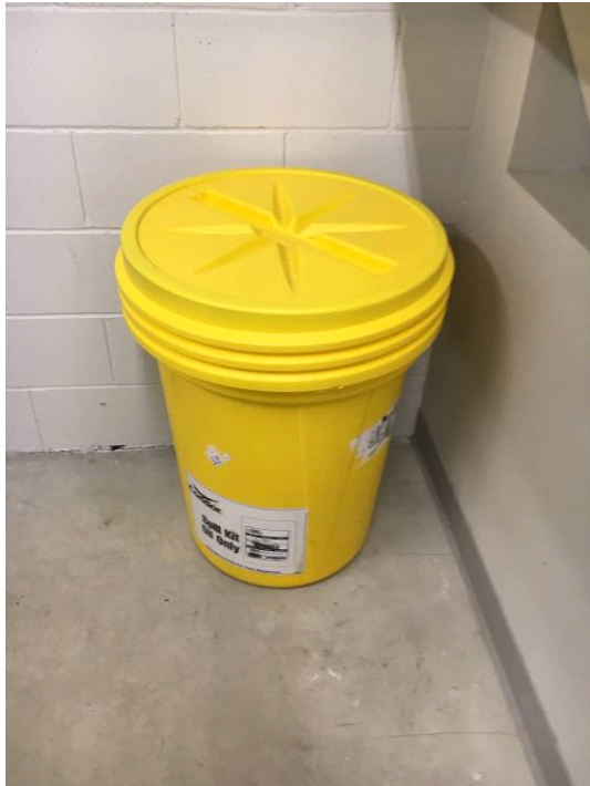
Figure B7. Unbraced Fluid Storage Container, in Room 306
