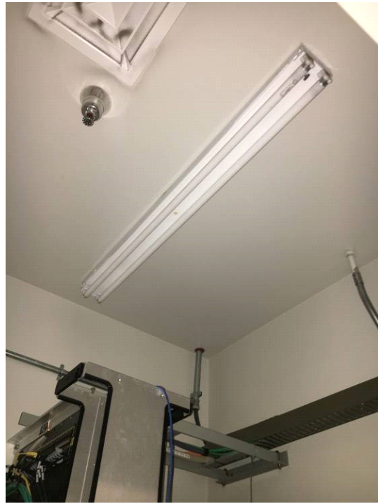
Figure B2. Light Fixture without Lens Cover, in Room 112A
