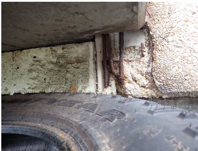
Vehicle Shop, West Man Door, Landing Ledger Figure B- 8
