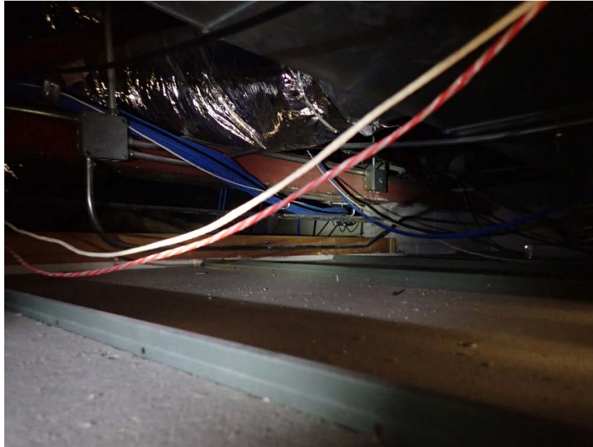
Room 368-369, Top of Wall Unrestrained Figure B- 45
