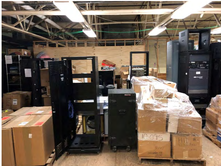
Mezzanine 238, Tall Narrow Contents Figure B- 78
