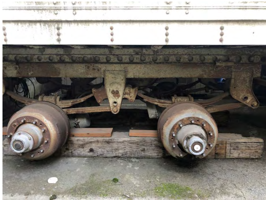
Vehicle Shop, West Bays Canopy, Base Support Figure B- 17
