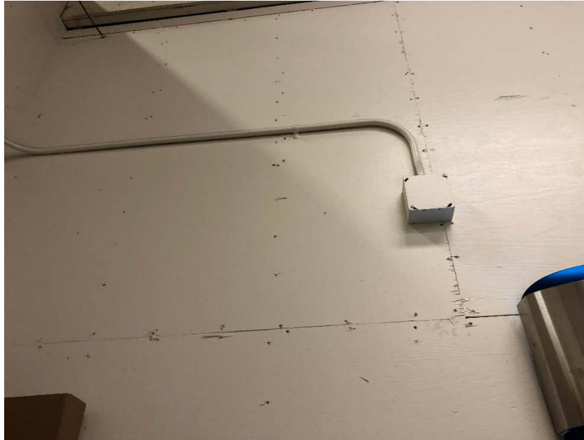
Room 116, Wood Shear Wall Figure B- 57
