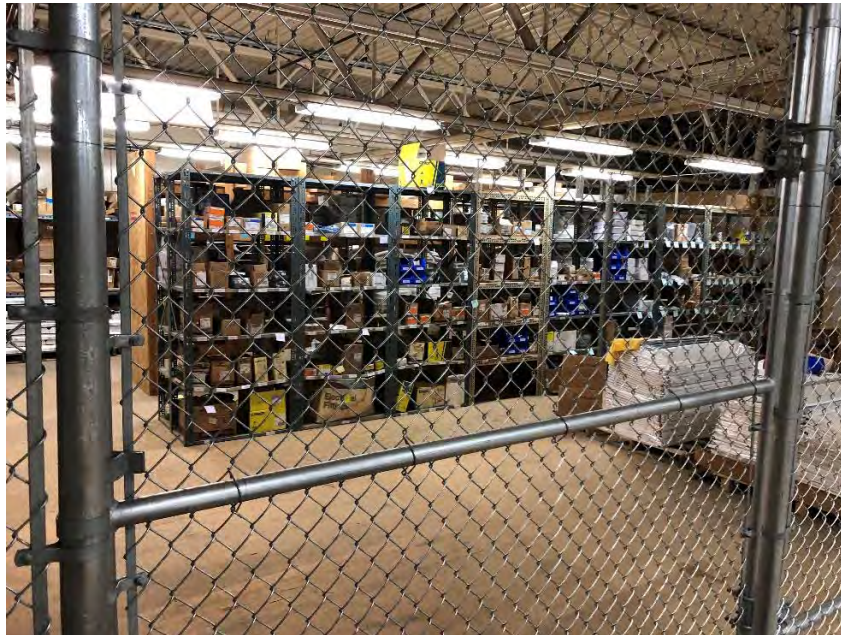
Mezzanine 238, Fall Prone Contents Figure B- 80
