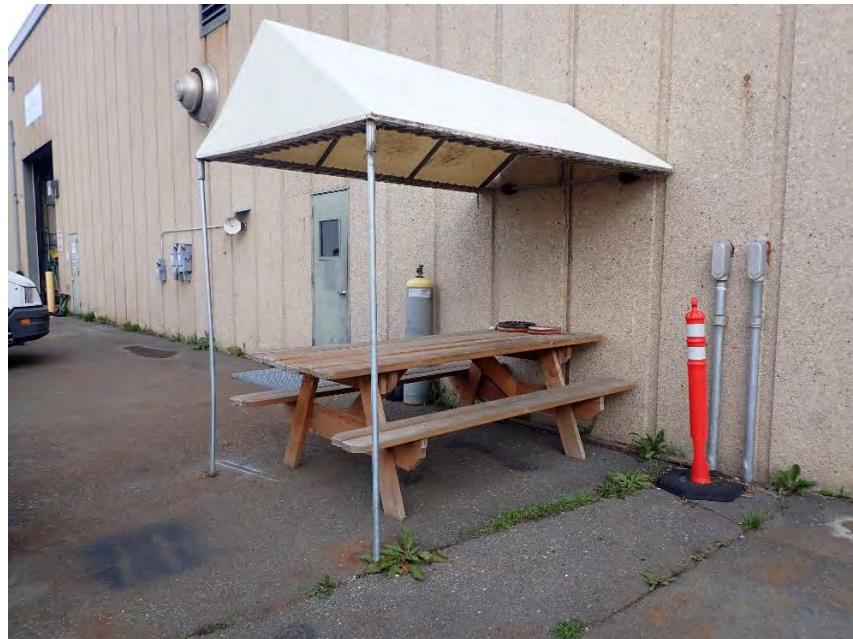
Vehicle Shop, South Canopy Figure B- 22
