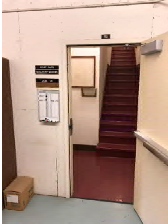
Corridor 190, Wood Shear Wall Figure B- 71
