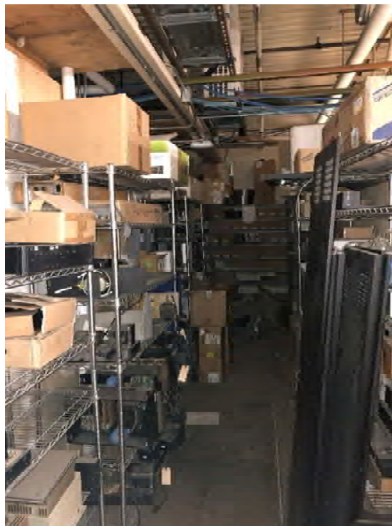
Mezzanine 238, Fall Prone Contents Figure B- 76
