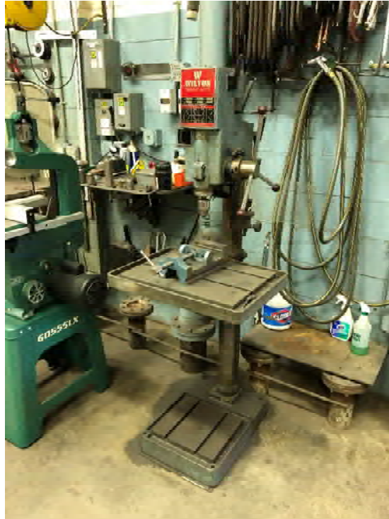
Welding Shop, Unrestrained Equipment Figure B- 93
