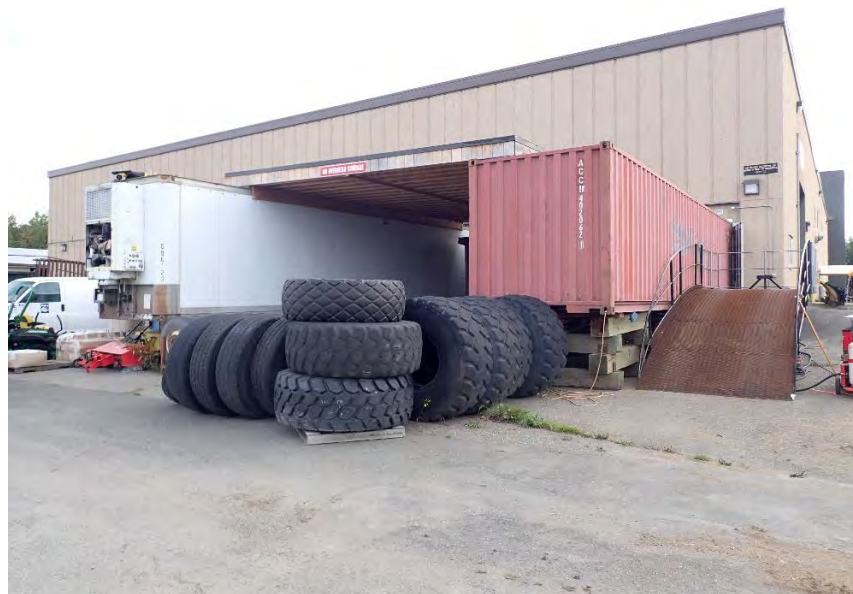
Vehicle Shop, West Bays Canopy Figure B- 12
