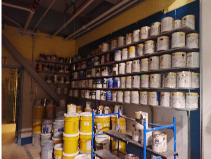
Paint Shop, Fall Prone Contents Figure B- 27
