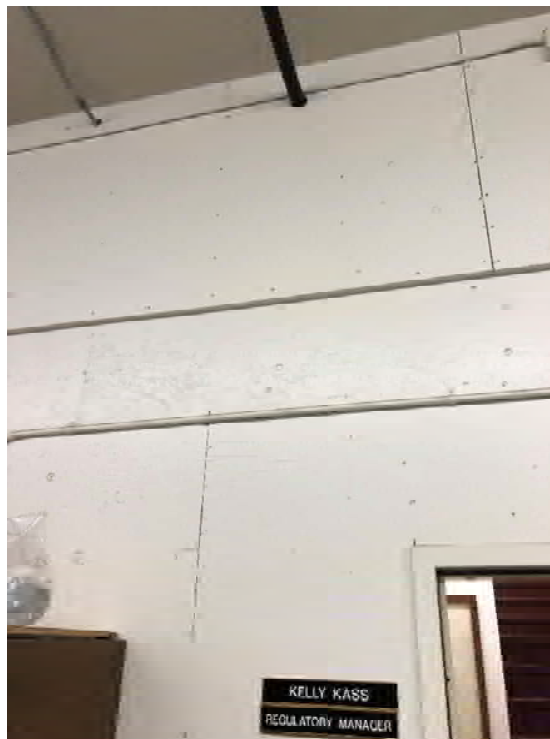
Corridor 190, Wood Shear Wall Figure B- 72
