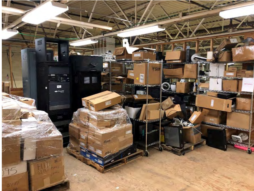
Mezzanine 238, Fall Prone Contents Figure B- 79
