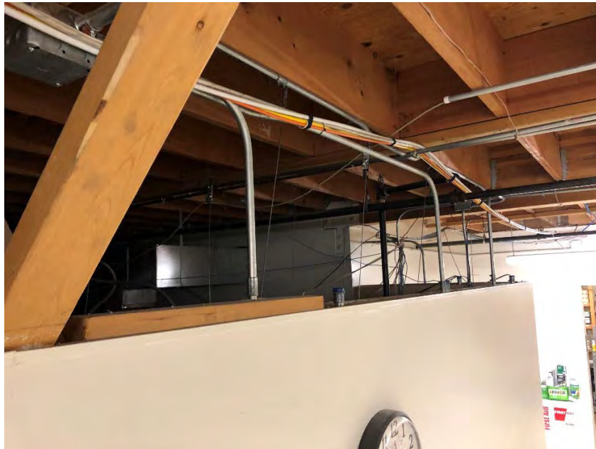
MCR Office, Ceilings Figure B- 70
