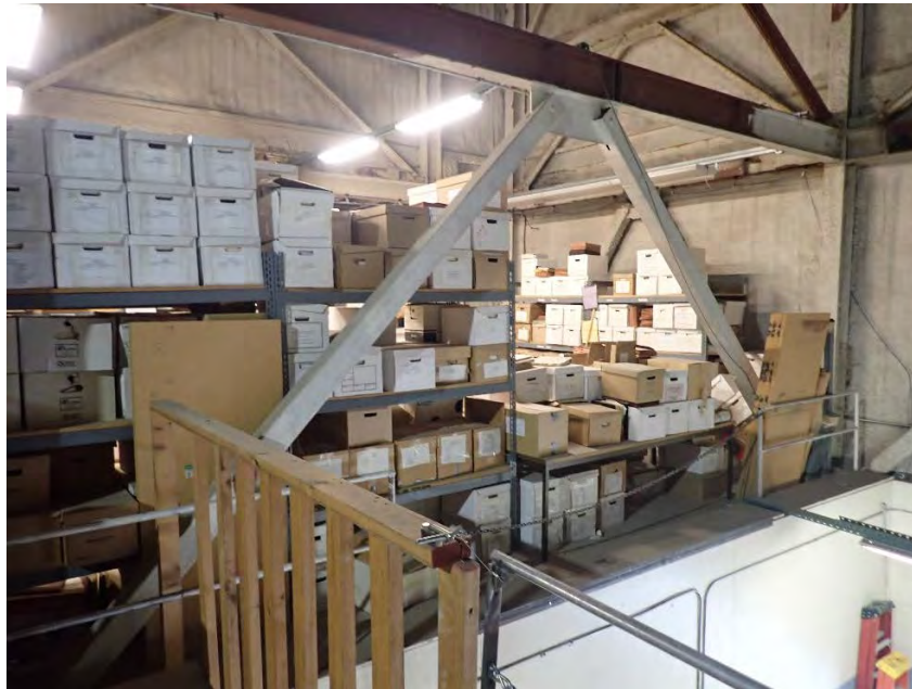
Room 223A, Fall Prone Contents Figure B- 44
