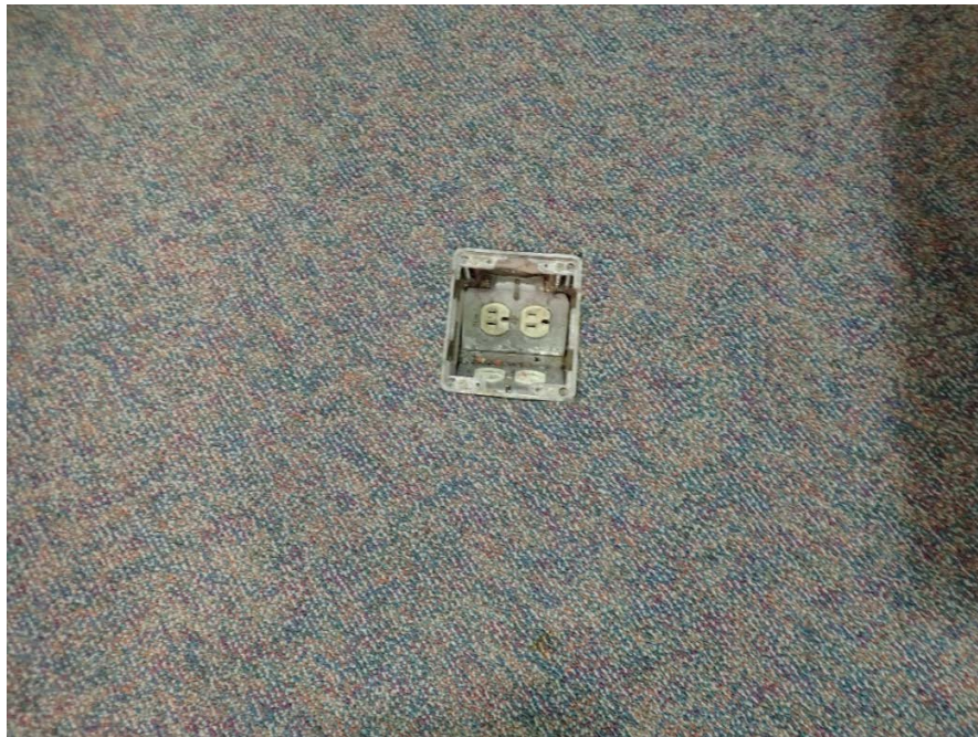
IMC, In Floor Receptacle without cover Figure B- 35
