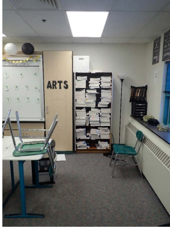
Room 132, Unrestrained Shelving Figure B- 23
