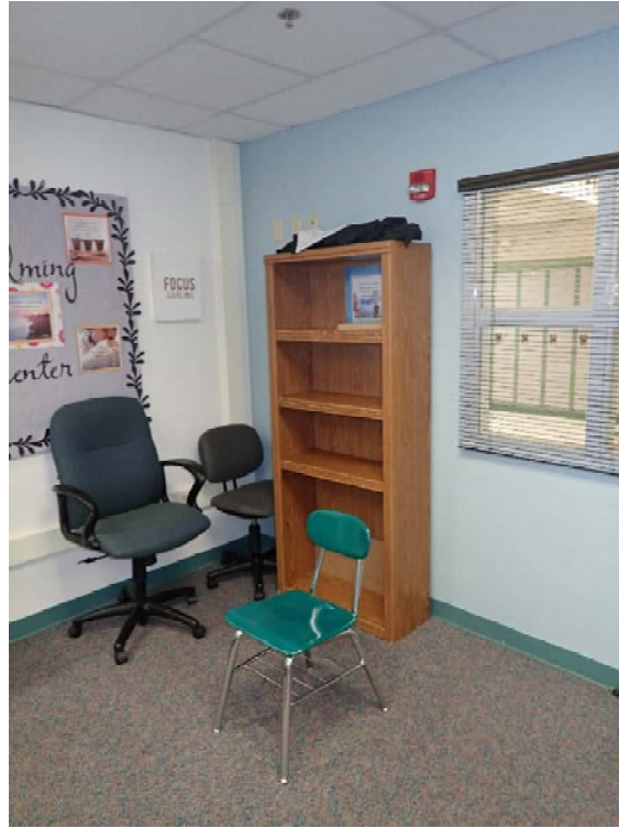
Room 119, Unrestrained Shelving Figure B- 31
