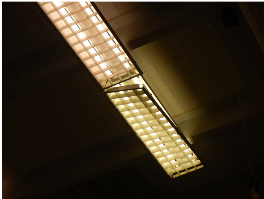
Auxiliary Gym, Lens Cover Detached Figure B- 4
