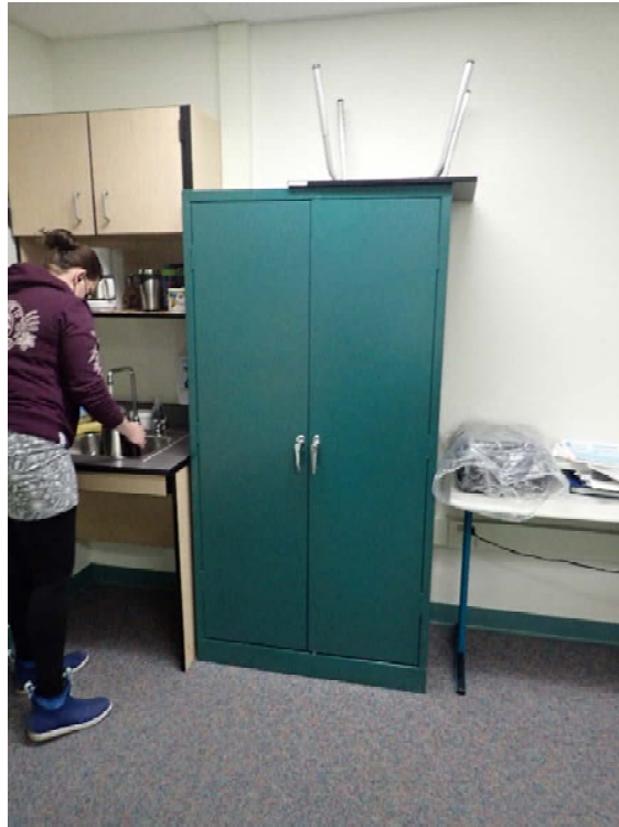
Room 131, Sprinkler w/ Insufficient Gap Figure B- 27
