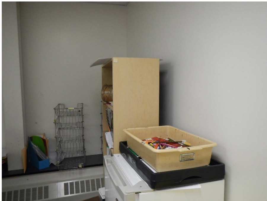
Room 137, Unrestrained Shelving Figure B- 13
