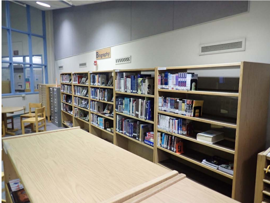
ICM, Unrestrained Shelving Figure B- 19
