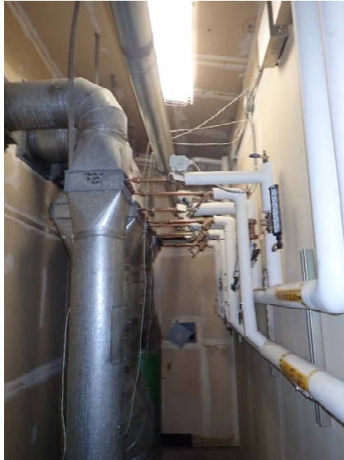
Room 201A, No Flexible Couplers Figure B- 32
