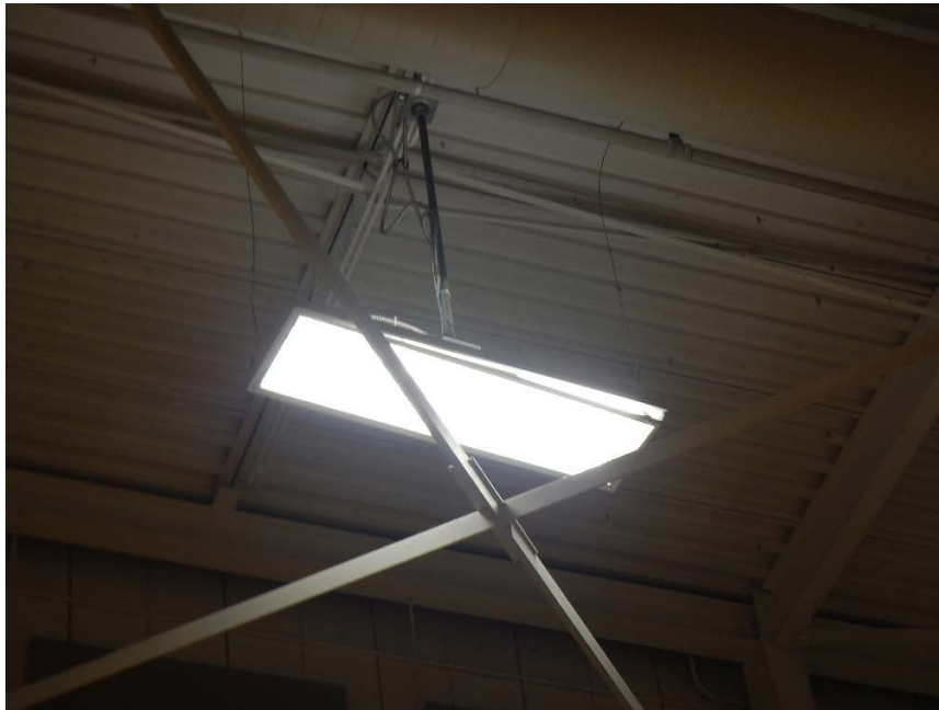
Main Gym, Lens Cover Detached Figure B- 3
