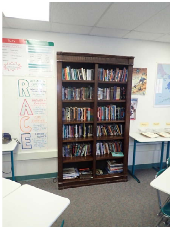
Room 130, Unrestrained Shelving Figure B- 28
