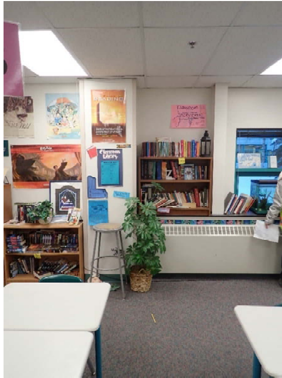
Room 129, Unrestrained Shelving Figure B- 29
