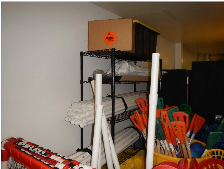
Room S07, Unrestrained Shelving Figure B- 16
