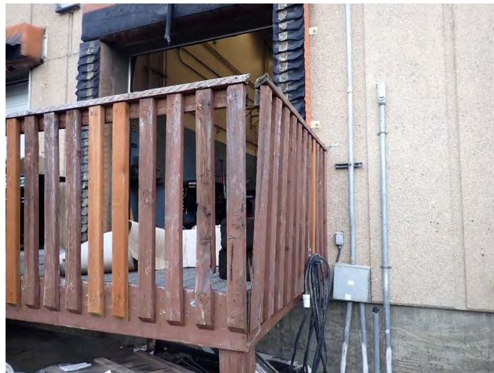
Vehicle Shop, West Bay Exit, Hand Rail Figure B- 2
