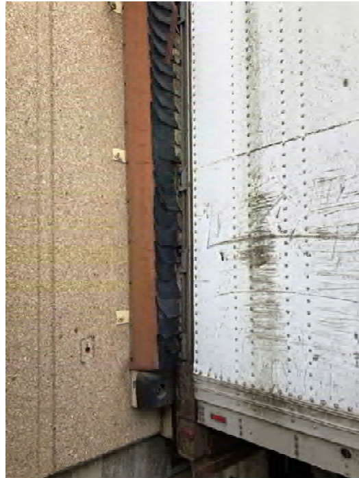
Vehicle Shop, West Bays Canopy, Conex to Main Structure B- 19
