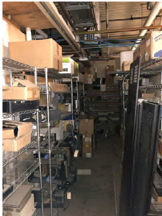
Mezzanine 238, Fall Prone Contents Figure B- 76
