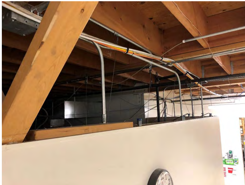
MCR Office, Ceilings Figure B- 70
