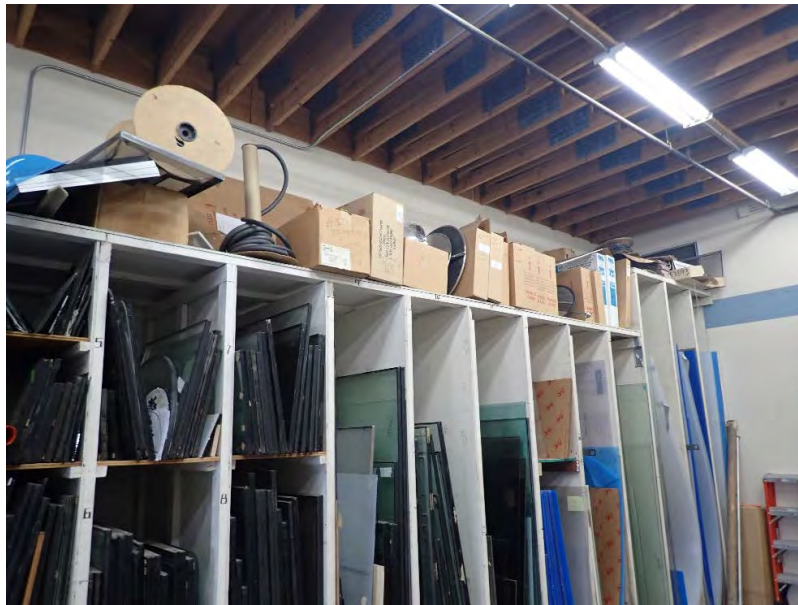
Glass Shop, Fall Prone Contents Figure B- 32
