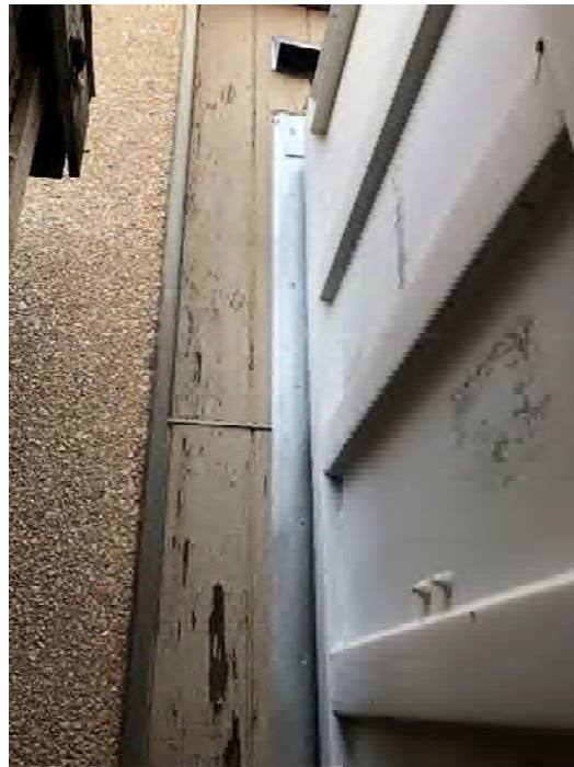
Vehicle Shop, West Bays Canopy, Conex to Main Structure B- 21
