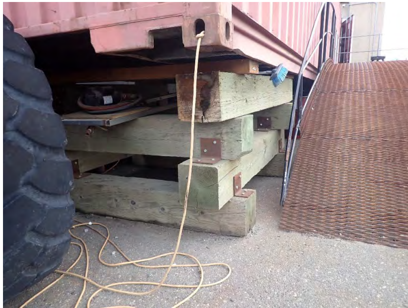
Vehicle Shop, West Bays Canopy, Base Support Figure B- 13
