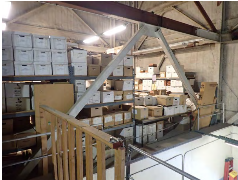
Room 223A, Fall Prone Contents Figure B- 44
