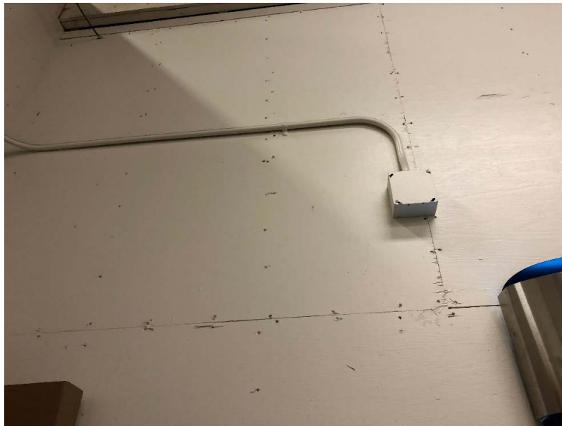
Room 116, Wood Shear Wall Figure B- 57
