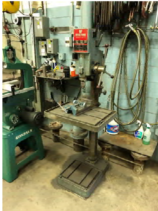
Welding Shop, Unrestrained Equipment Figure B- 93
