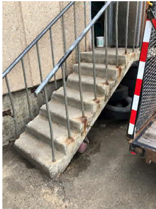
Vehicle Shop, West Man Door, Stairs Figure B- 5
