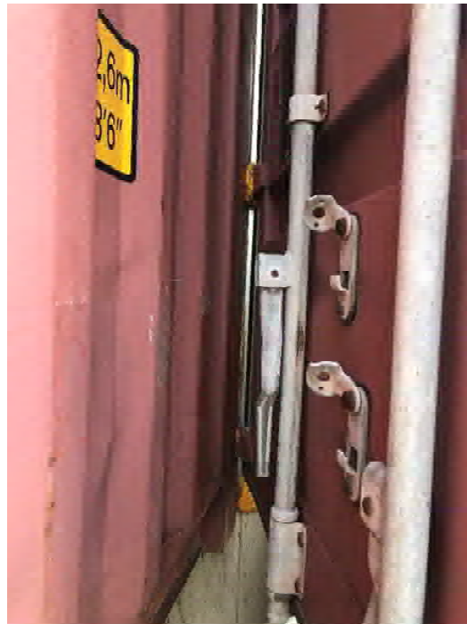
Vehicle Shop, West Bays Canopy, Conex to Main Structure B- 15
