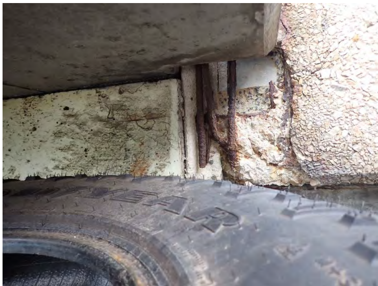
Vehicle Shop, West Man Door, Landing Ledger Figure B- 8
