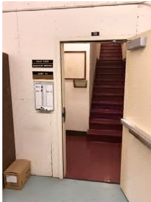
Corridor 190, Wood Shear Wall Figure B- 71
