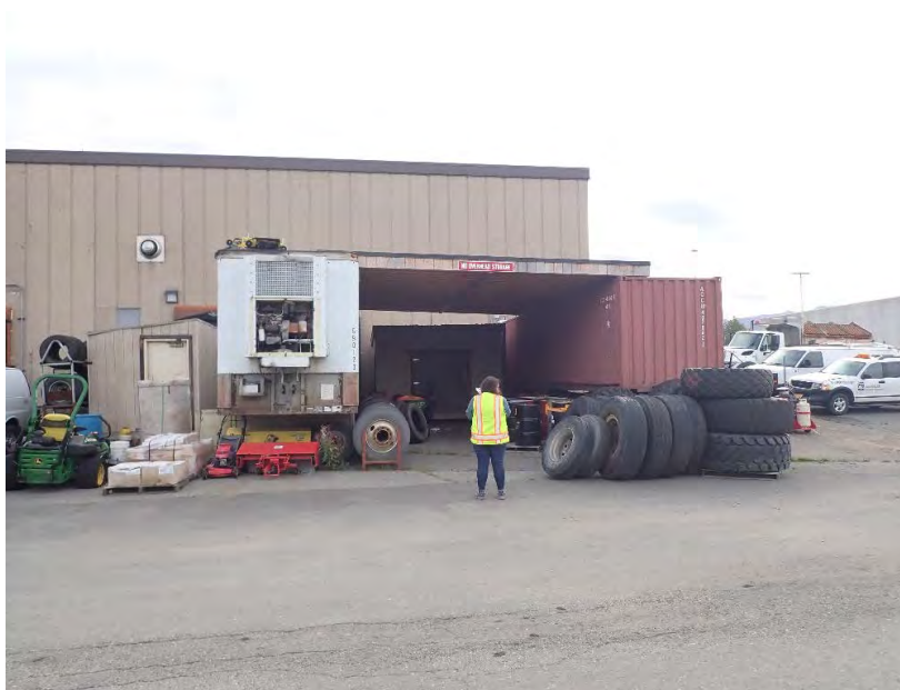
Vehicle Shop, West Bays Canopy Figure B- 11
