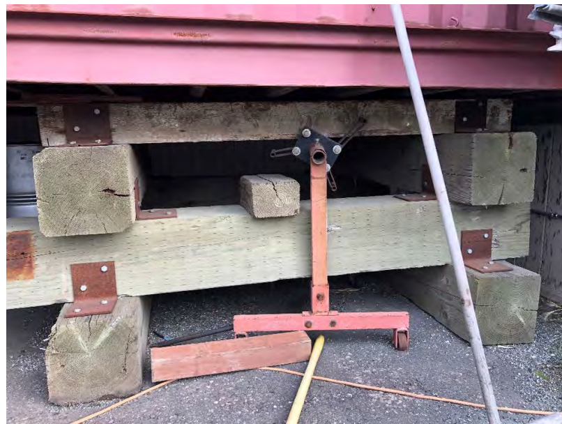
Vehicle Shop, West Bays Canopy, Base Support Figure B- 18
