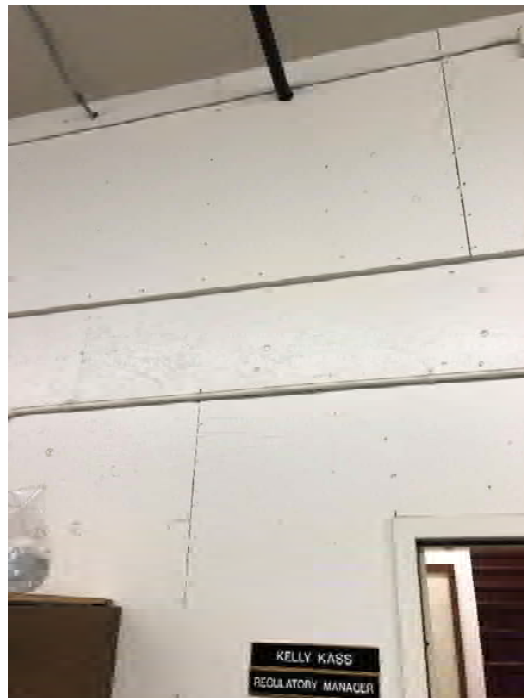
Corridor 190, Wood Shear Wall Figure B- 72
