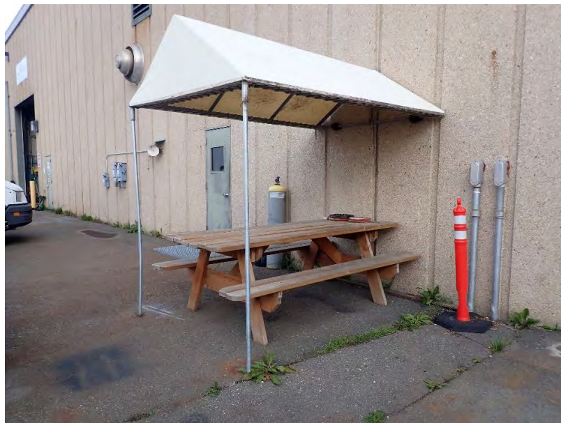
Vehicle Shop, South Canopy Figure B- 22
