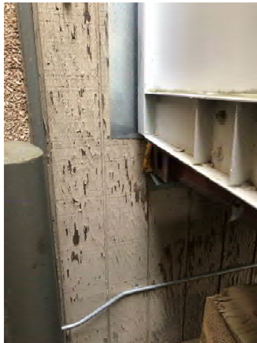
Vehicle Shop, West Bays Canopy, Conex to Main Structure B- 20
