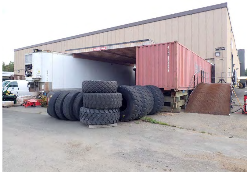
Vehicle Shop, West Bays Canopy Figure B- 12
