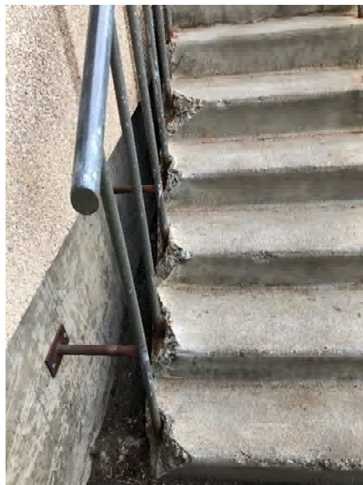
Vehicle Shop, West Man Door, Stair Attachment Figure B- 6
