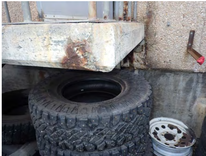
Vehicle Shop, West Man Door, Cantilever Landing Figure B- 7
