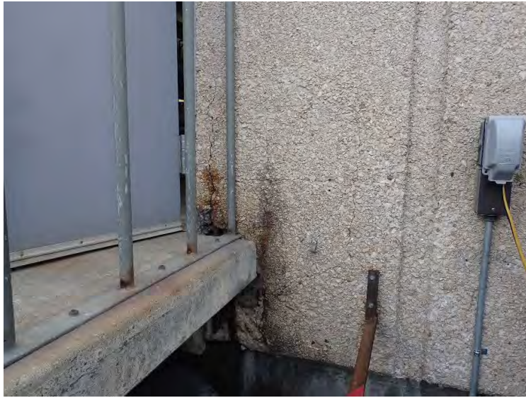
Vehicle Shop, West Man Door, Landing Ledger Figure B- 9
