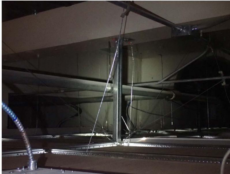
MCR Storage, Proper Integrated Ceiling Figure B- 33
