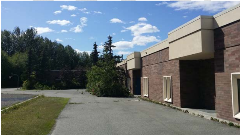
Existing exit door alcoves with overhang
