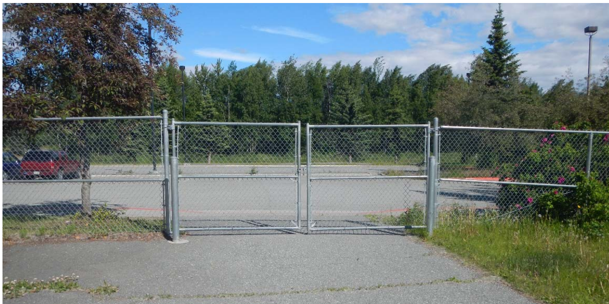
The existing gates on the north and south side of the school do not meet the minimum 20' width requirement for fire lanes.
