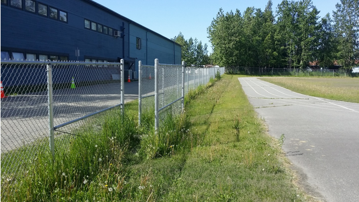
Perimeter fence and pedestrian pass through west of the track with lawn strip and elevation change between properties
