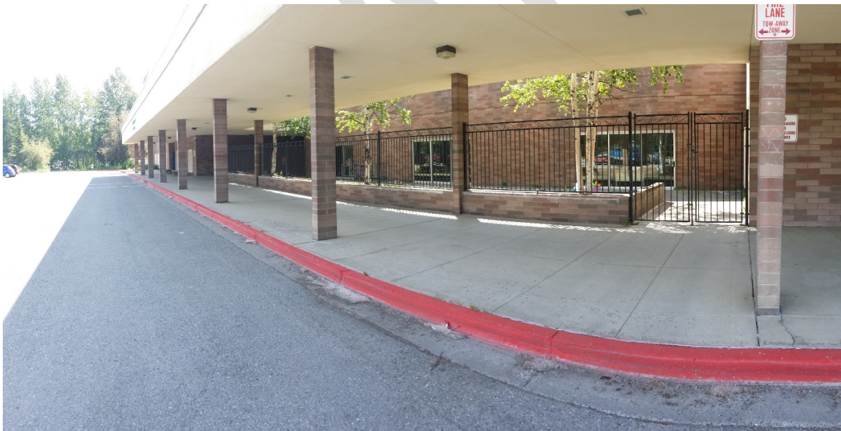
Bus and parent drop-off area at east canopy, looking southwest towards Courtyard and Main Entry
