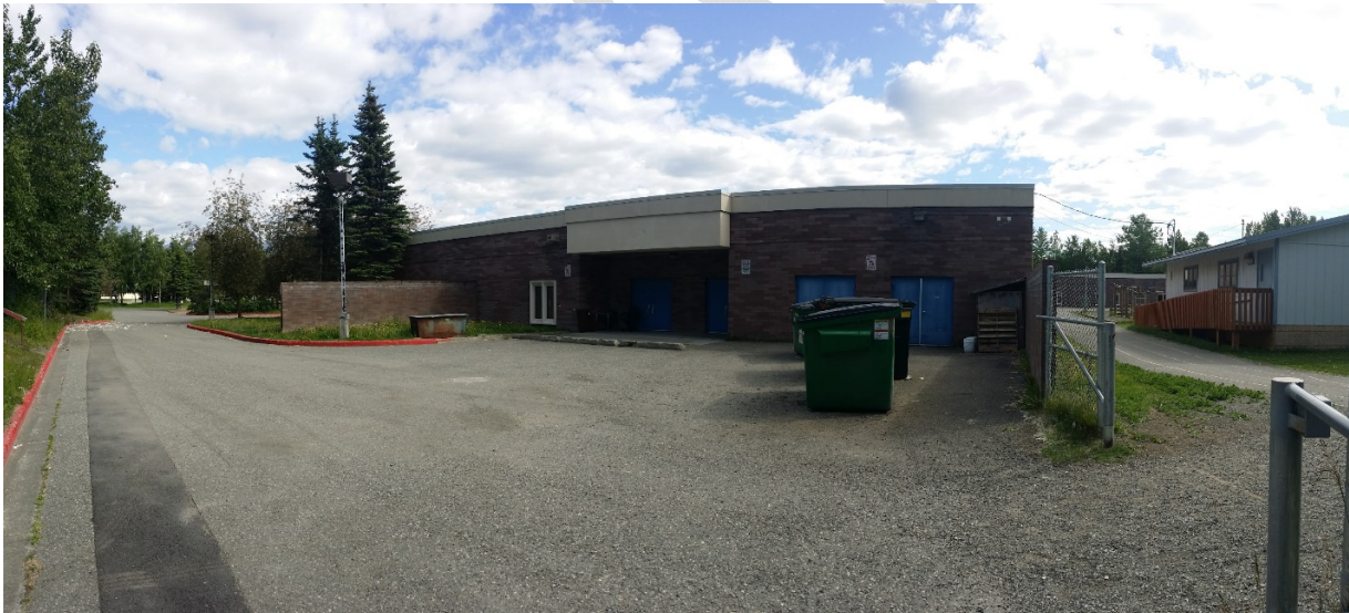
Service area, fire lane and fire lane access gate at north end of school with gravel paved segment connecting to asphalt track and relocatable
