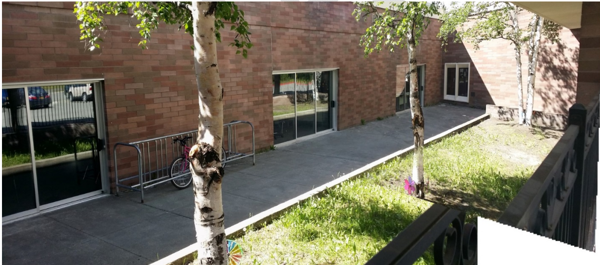
Main entry Courtyard area with damaged Paper Birch and lawn planter
