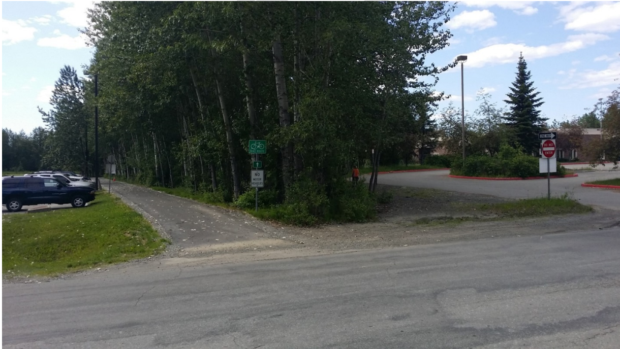
Recently rehabilitated Chester Creek Trail segment terminates at west edge of Nichols Street near Whaley south exit drive
