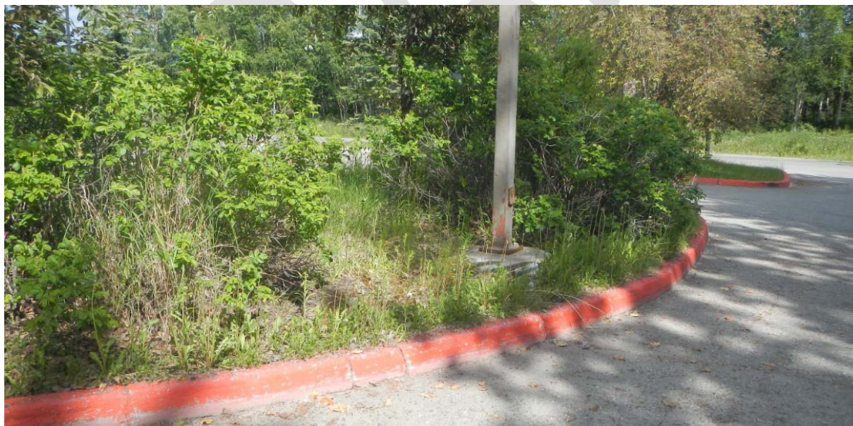
Overgrown Vegetation in the Parking Lot Island blocking Vehicle Site Distance
