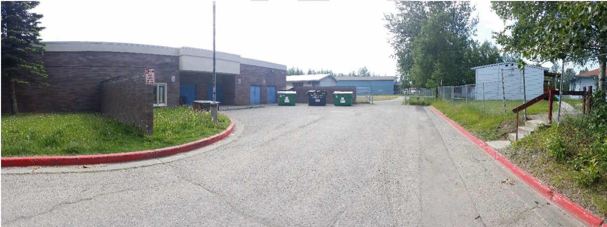
Service area with vehicle gates and pedestrian opening in perimeter fence with stairs and handrail in poor condition
