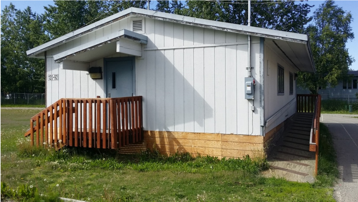
Existing relocatable classroom in north recreation area without paved accessible route
