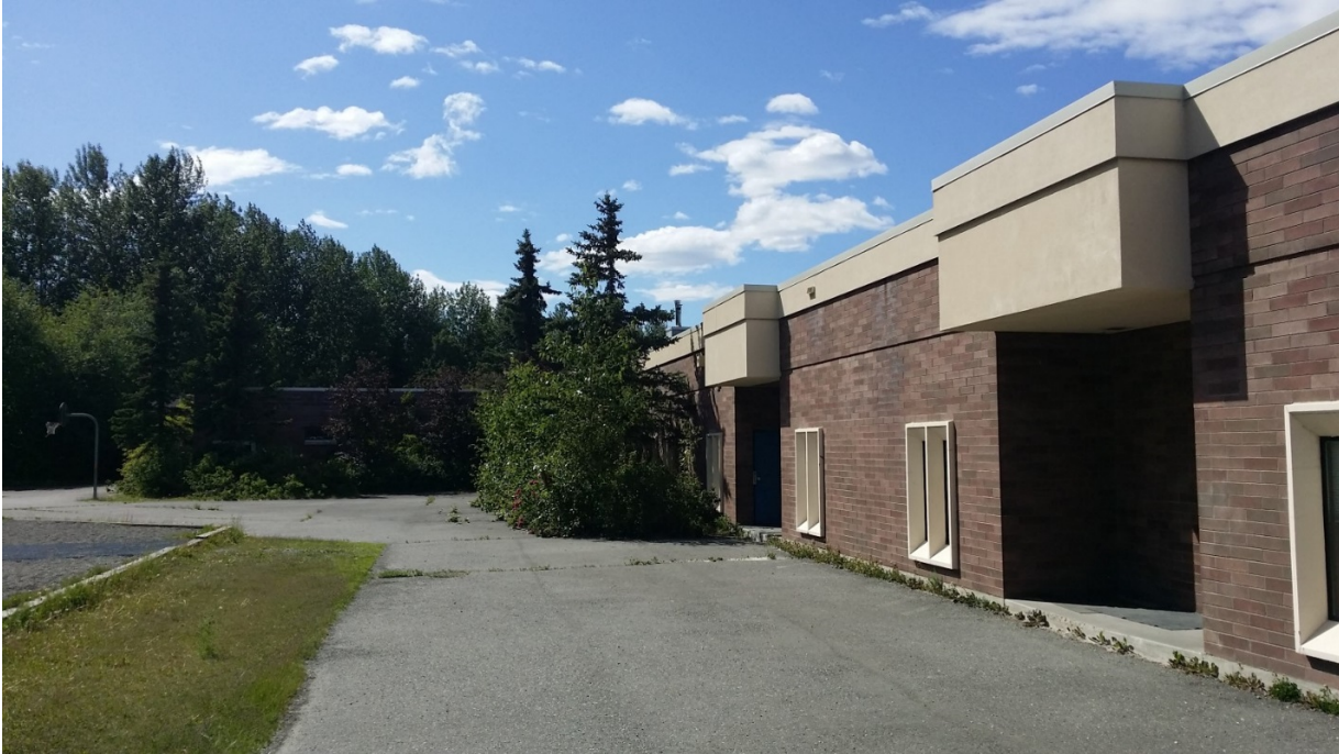
South exterior entries with step down to asphalt pavement and overgrown vegetation
