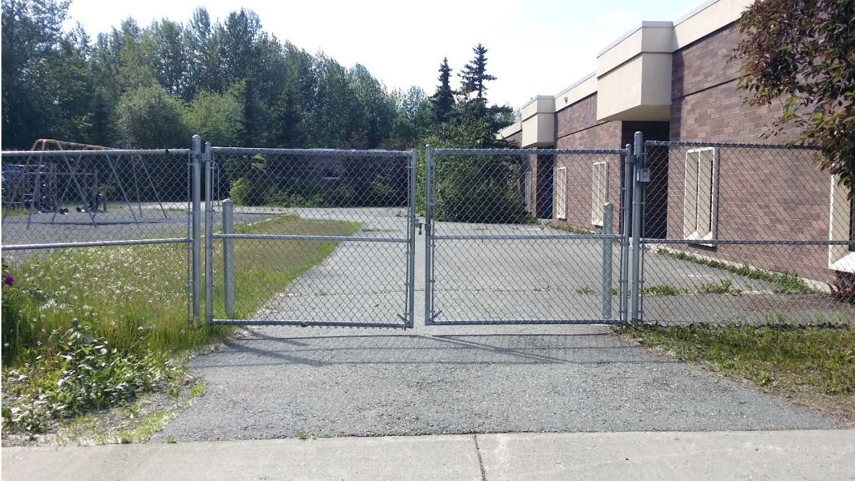
Fire Lane access gate at south recreation area
