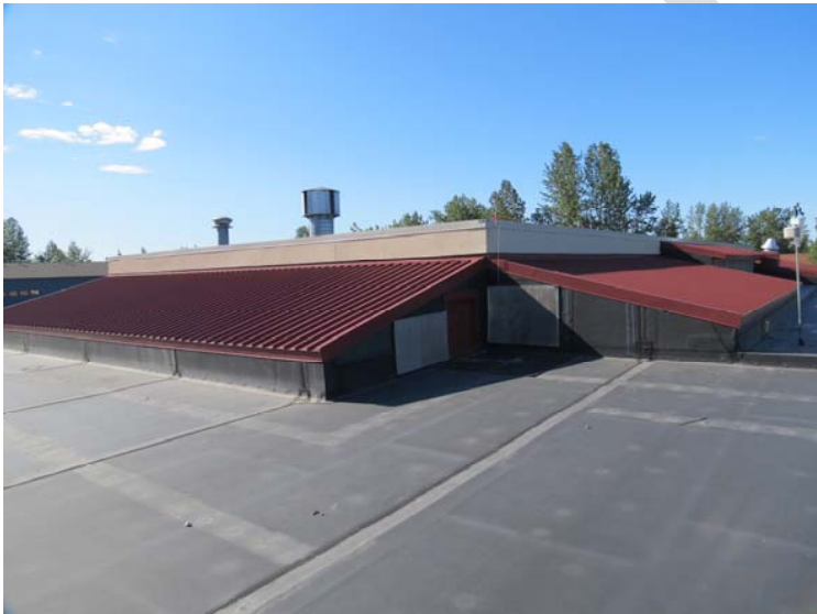
Existing Fan room over the original building
