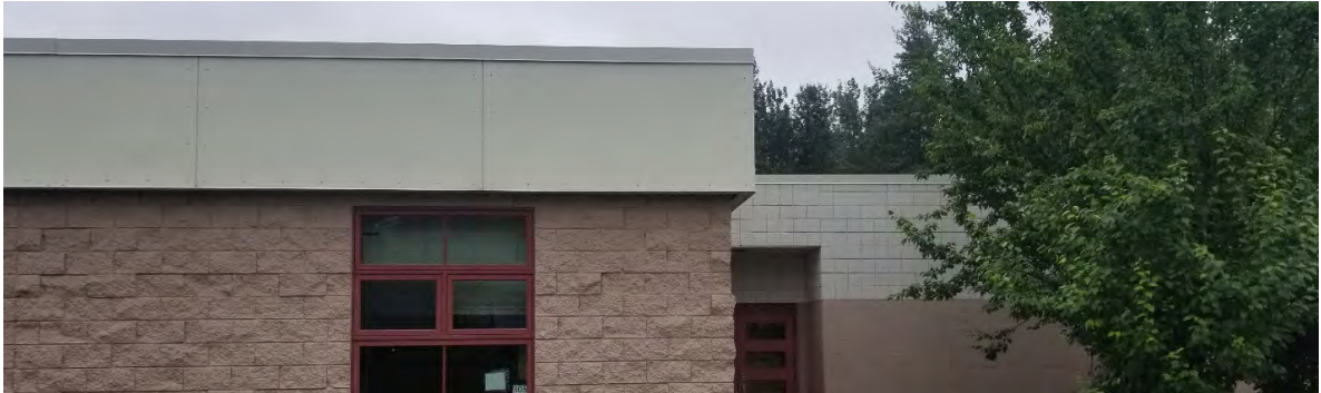
Figure 34 - Exterior cladding at top of CMU wall, typical at 1999 additions.
