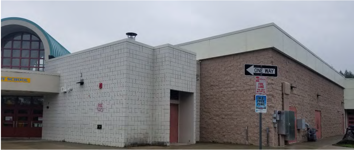
Figure 14 – Boiler room and storage, Southwest elevation.
