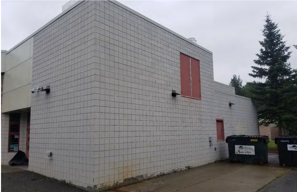
Figure 17 – Multi-purpose room and south mechanical penthouse.
