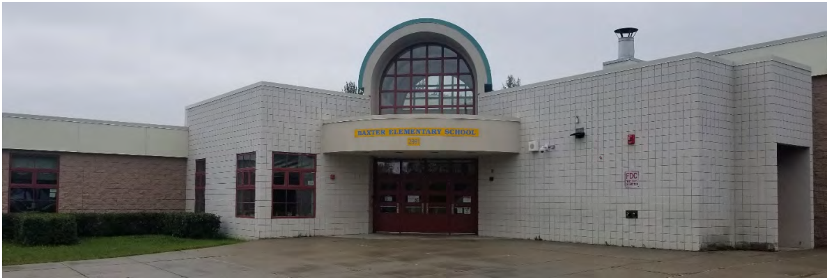
Figure 13 – Main entrance to the school, Southwest elevation.
